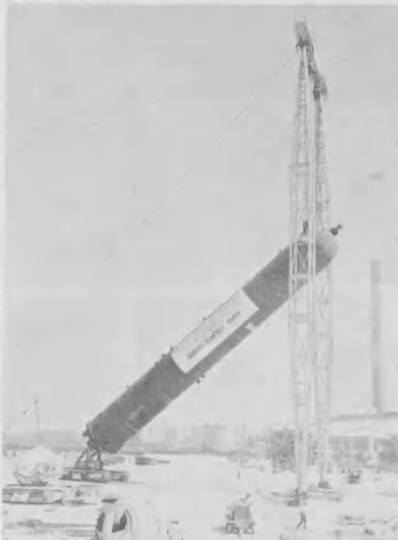
640-ton, 135 ft. high reactor for Heavy Vacuum Oil Hydrofiner.
